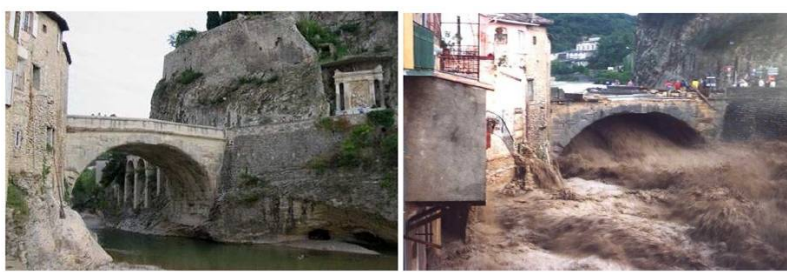
Figure 1. L'Ouvèze at Vaison la Romaine; the flow of this river of Provence has been able to increase from 0.1 \text{ m}^3/\text{s} - left photo, summer 1990- to nearly 1200 \text{ m}^3/\text{s} - right photo, September 22, 1992- this for an average annual flow close to 6 \text{ m}^3/\text{s} . [© EDF DTG]
