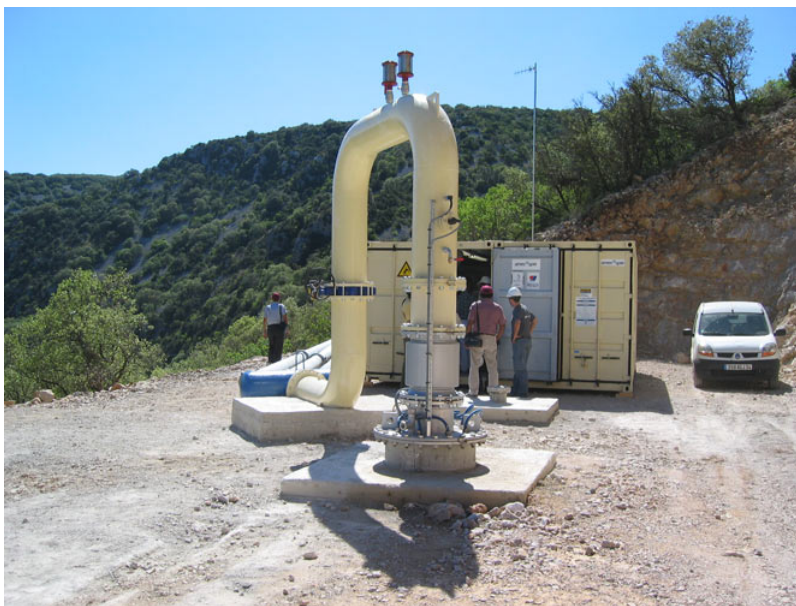
Figure 11. High flow pumping test, source of the Cent-Fonts (Hérault). [© M. Bakalowicz]
