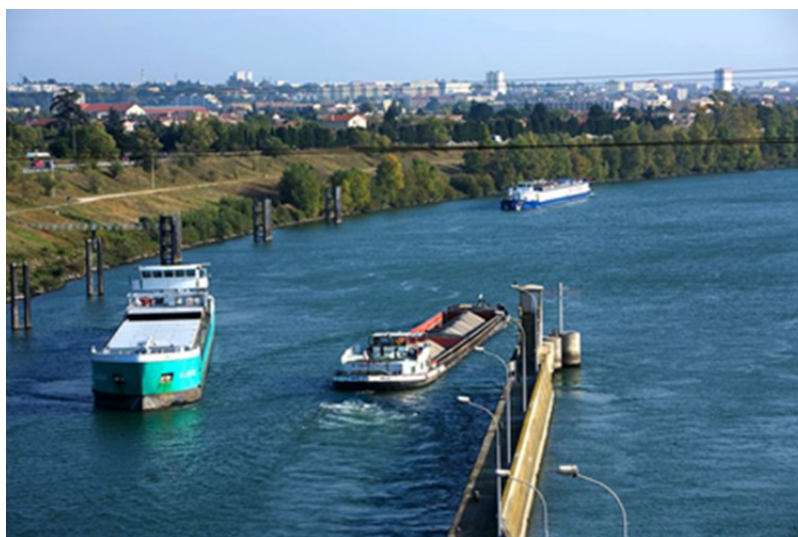
Figure 5. Lock entrance [Source: © Camille Moirenc]
