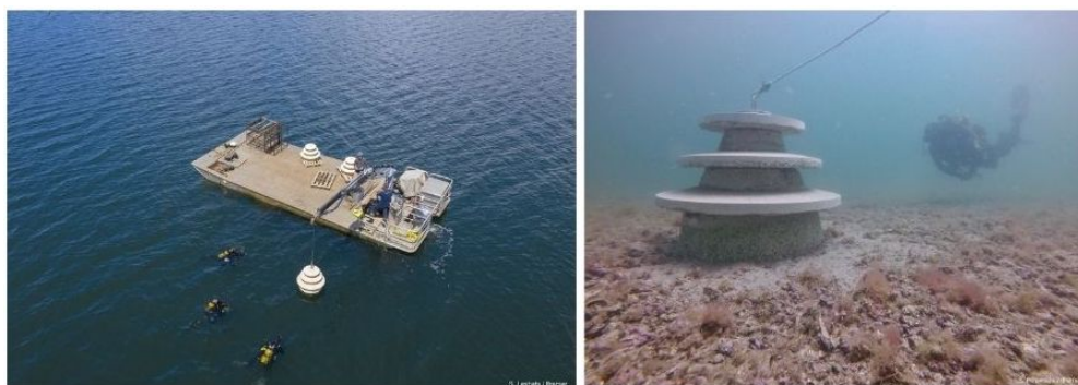
Figure 13. Restoring the former oyster beds of the past: implantation of concrete shell reefs in order to favour recruitment and revitalise the flat oyster populations of the Roz bank in Brest bay and the Penthièvre bank in Quiberon bay. [Source: © IFREMER / Stéphane Lesbats (left) & Stéphane Pouvreau (right)]
