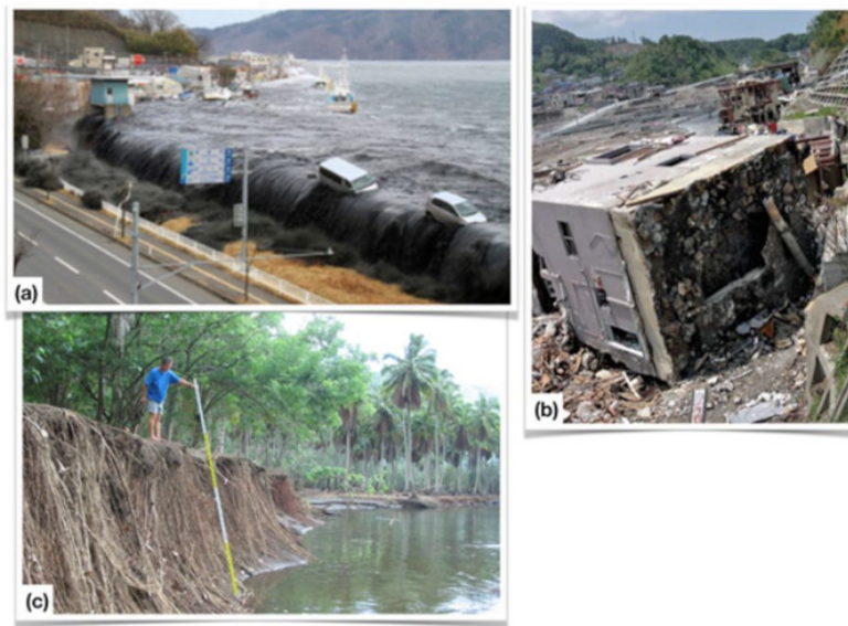
Figure 4. (a) Arrival of the 2011 tsunami in Miyako Bay, and overflow of the protective wall (source: Flickr) (b) Three-storey building overturned by the tsunami in Onagawa (source: International Tsunami Information Center ) (c) Impact of the 2011 tsunami in Taipivai Bay at Nuku-Hiva in the Marquesas Islands (French Polynesia), the tsunami widened the riverbed by digging the banks to a height of about 3 m. [Source: © CEA]
