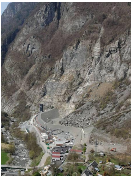
Figure 8. Merlon de protection [Source : Gavet, photo Sage]
