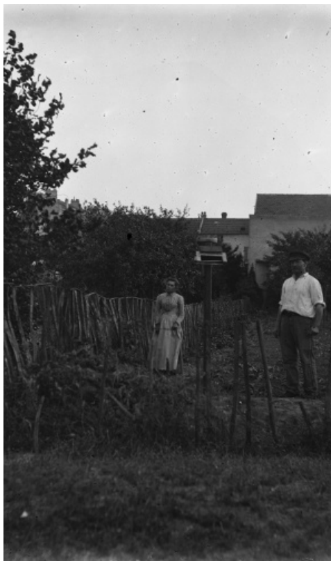
Figure 10. Rainfall observation in Noisy le Sec in 1897. [© Météo-France]
