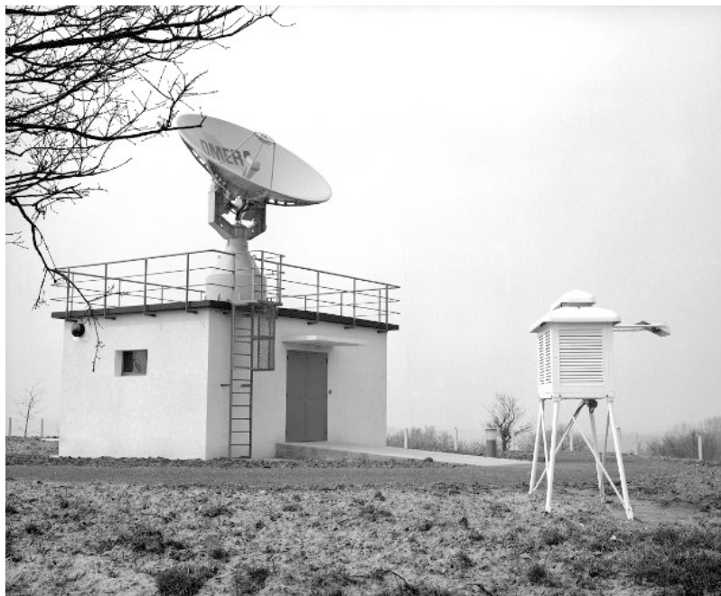
Figure 16. One of the first French precipitation radars, the Melodi, in Dammartin, in 1974. [© Météo-France]
