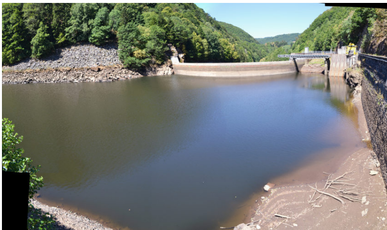
Figure 6. Vaussaire dam during low water periods. The tidal range can also be several metres under certain conditions. This exposure to atmospheric conditions can promote certain reactions (oxidation in particular) within the sedimentary matrix. [© A. Courtin-Nomade]
