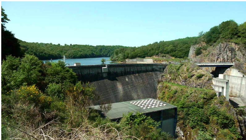
Figure 3. Example of a weight dam (Rochebut) used in hydroelectricity. [© A. Courtin-Nomade]
