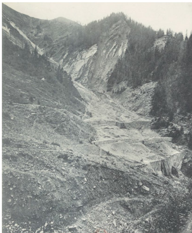
Figure 5. Dams retaining moraine deposits from the headwaters: Ravin des Arandellys, a tributary of the Griez River that flows into the Arve River downstream of the EDF Houches hydro-electricity dam (74). [Source: Waters and Forests 1911 [20]]
