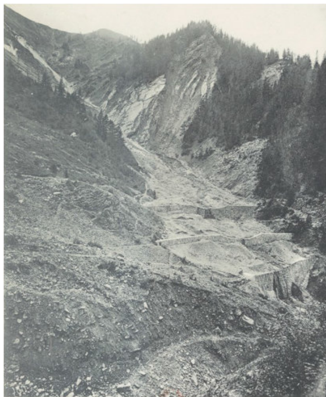
Figure 5. Dams retaining moraine deposits from the headwaters: Ravin des Arandellys, a tributary of the Griez River that flows into the Arve River downstream of the EDF Houches hydro-electricity dam (74). [Source: Waters and Forests 1911 [201]]
