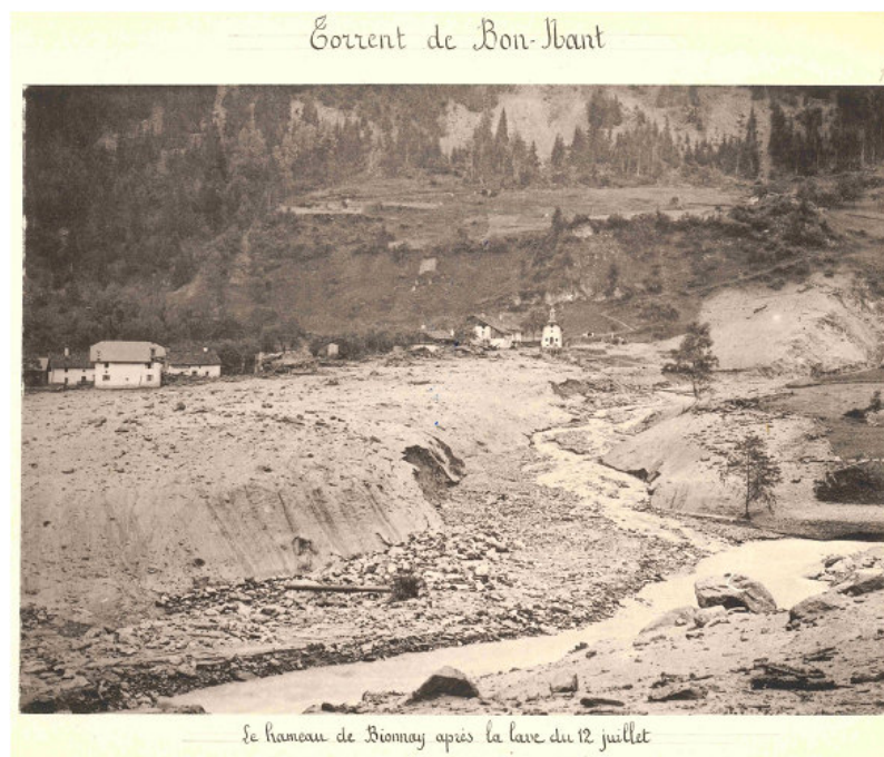
Figure 4. Hamlet of Bionnay ravaged by the rupture of the Tête Rousse glacier lake outburst flood and the debris flow that formed downstream. Catastrophe which caused 175 deaths in 1892. [© Kuss [191]]
