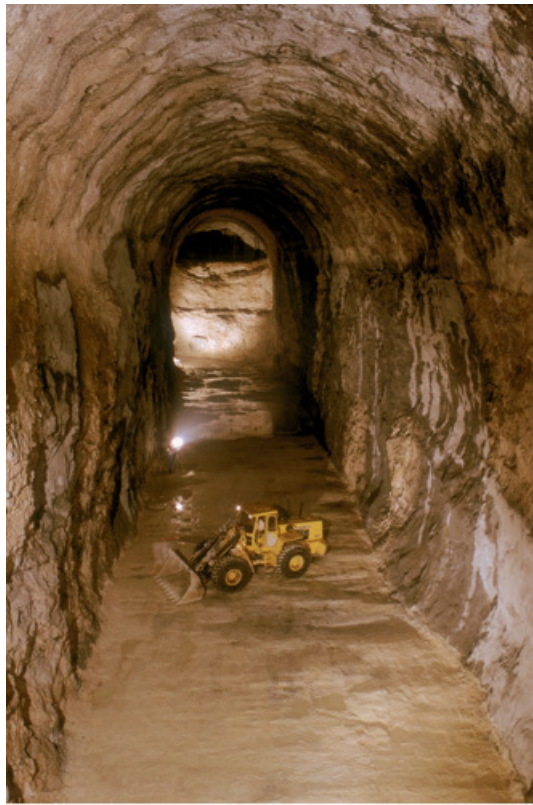
Figure 3. Digging an unlined storage gallery at Lavéra. [© Geostock Photo Library]
