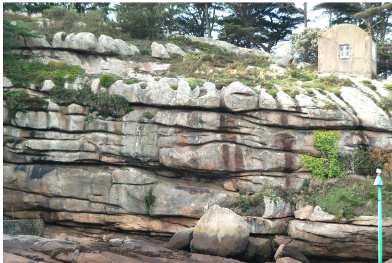
Figure 4. Example of fractures (subhorizontal) within the fractured horizon of a granite. The house on the top right has a maximum height of about 3 m. Ploumanac'h, Côtes d'Armor, France. [© R. Wyns]
