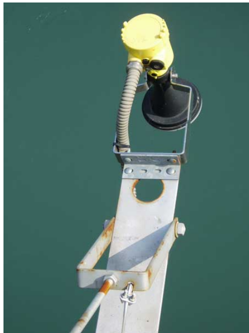
Figure 5. Level measurement by emerged radar. [© EDF DTG]
