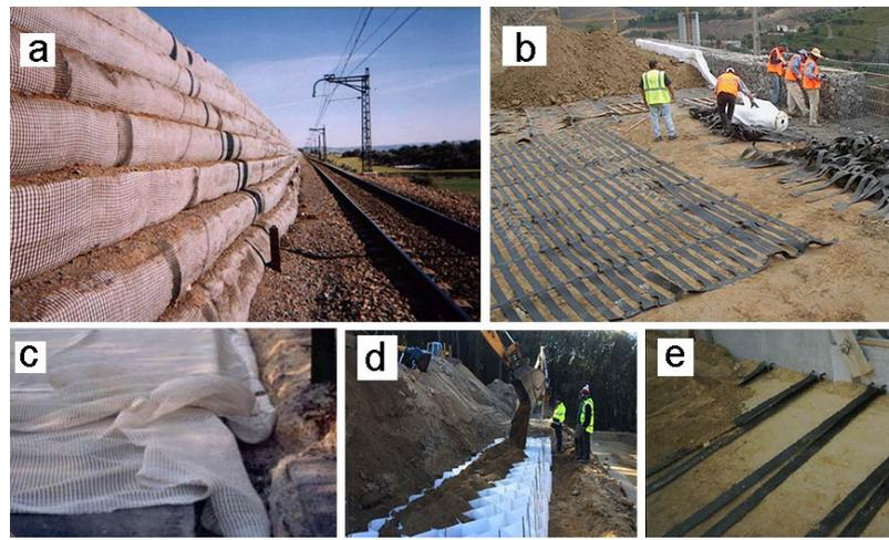
Figure 2. Reinforcement of support structures. (a) Geosynthetically reinforced wall; (b) Geogrid reinforcement; (c) Geotextile web reinforcement; (d) Cell structure reinforcement (Armatex process[1]) and (e) Geotextile band reinforcement.
