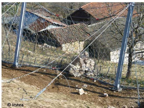
*Figure 9. Deformable nets, Ripailler. [Source: IRSTEA]*
