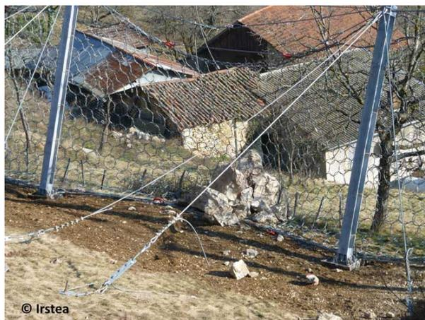
*Figure 9. Deformable nets, Ripailler. [Source: IRSTEA]*
