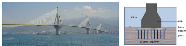
Figure 7. The Rion-Antirion cable-stayed viaduct, made of reinforced concrete and steel, put into service in 2004, crosses the Strait of Patras in Greece, very seismic, by 65 m of water, whose seabed consists of a thick layer mainly clayey and soft. 2883 m long, based on 4 piers with a diameter of 90 m and a maximum span between piles of 560 m, it combines preventive measures. The clay under the piers is reinforced by a 30 m long forest of metal piles, which prevents a rotation of the soil-pier assembly. These piles are surmounted by a fusible granular layer (basalt blocks), allowing relative horizontal displacement (irreversible sliding) of piers during major earthquakes. On the left, view of the viaduct. On the right, the principle of improving the foundation soil. [Left, source: By David Monniaux (Own work)] [GFDL ( http://www.gnu.org/copyleft/fdl.html ), CC-BY-SA-3.0 ( http://creativecommons.org/licenses/by-sa/3.0/ ) or CC BY-SA 2.0 en ( http://creativecommons.org/licenses/by-sa/2.0/fr/deed.en )], via Wikimedia Commons. [Right, © Marc Boulon]
