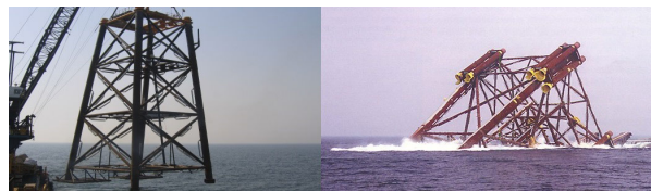
Figure 2. On the left, one of the jackets elements supporting an offshore platform, up to 300 m of water, size and weight comparable to those of the Eiffel Tower. On the right, jacket equipped with flotation ballasts towed on site; pile (diameter 2 m, length 50 to 100 m) guide sleeves for nailing on the sandy seabed. [Source: A. Puech, 2008, Cours de géotechnique marine, ENSHMG]
