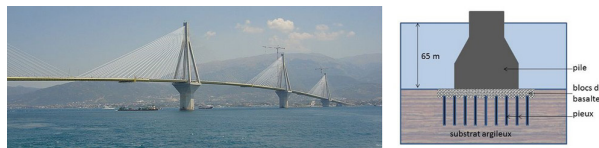
Figure 7. The Rion-Antirion cable-stayed viaduct, made of reinforced concrete and steel, put into service in 2004, crosses the Strait of Patras in Greece, very seismic, by 65 m of water, whose seabed consists of a thick layer mainly clayey and soft. 2883 m long, based on 4 piers with a diameter of 90 m and a maximum span between piles of 560 m, it combines preventive measures. The clay under the piers is reinforced by a 30 m long forest of metal piles, which prevents a rotation of the soil-pier assembly. These piles are surmounted by a fusible granular layer (basalt blocks), allowing relative horizontal displacement (irreversible sliding) of piers during major earthquakes. On the left, view of the viaduct. On the right, the principle of improving the foundation soil. [Left, source: By David Monniaux (Own work)] [GFDL ( http://www.gnu.org/copyleft/fdl.html ), CC-BY-SA-3.0 ( http://creativecommons.org/licenses/by-sa/3.0/ ) or CC BY-SA 2.0 en ( http://creativecommons.org/licenses/by-sa/2.0/fr/deed.en )], via Wikimedia Commons. [Right, © Marc Boulon]
