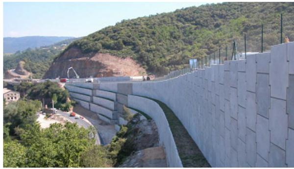
Figure 6. A high retaining wall made of "reinforced earth wall". Each wall level consists of joined reinforced concrete "scales" anchored by friction in the upstream embankment by means of metal rods. The backfill is built as the wall is erected. This technique makes it possible to create aesthetic, stable, sub-vertical and draining walls. [Source: E. Lucas, P. Sery, A. Tigoulet, D. Brancaz, 2008, *Les ouvrages récents de grande hauteur en sol renforcé*, *Compte rendu JNGG 2008*, Nantes]
