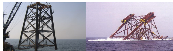
Figure 2. On the left, one of the jackets elements supporting an offshore platform, up to 300 m of water, size and weight comparable to those of the Eiffel Tower. On the right, jacket equipped with flotation ballasts towed on site; pile (diameter 2 m, length 50 to 100 m) guide sleeves for nailing on the sandy seabed. [Source: A. Puech, 2008, Cours de géotechnique marine, ENSHMG]
