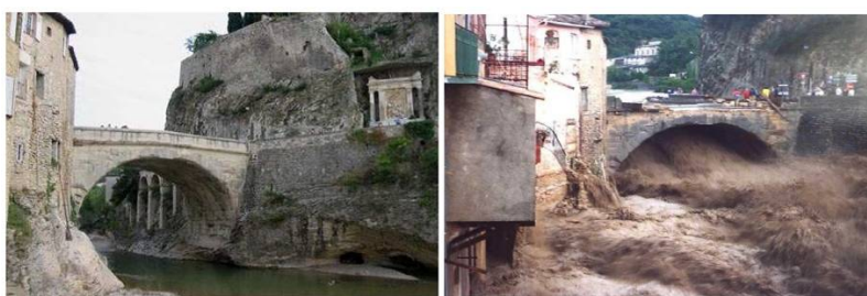
Figure 1. L'Ouvèze at Vaison la Romaine; the flow of this river of Provence has been able to increase from 0.1 m 3 /s - left photo, summer 1990- to nearly 1200 m 3 /s- right photo, September 22, 1992- this for an average annual flow close to 6 m 3 /s. [© EDF DTG]
