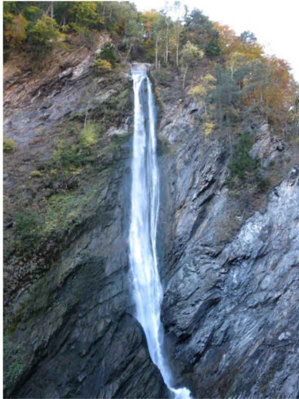
*Figure 7. Downstream outlet of the tunnel bypassing a landslide on the Morel torrent (Aigueblanche, 73). The tunnel, drilled in the stable slope opposite the landslide, diverts the stream from the bottom of the landslide (located on the other side of the valley shown on the right of the photo) and prevents the stream from eroding the bottom of the unstable mass and loading itself with sediments that it would carry downstream over high stakes areas. [© G. PITON]*
