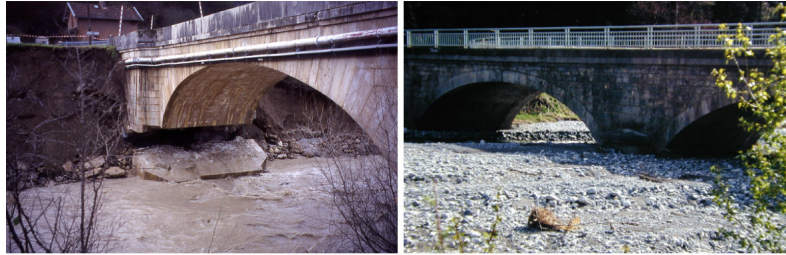
Figure 6. Two examples of the evolution of a river bed and its consequences on a bridge: on the left, the sinking of the bed can lead to destabilization of the structure, Pont des Chaines à Die. [©F. Liebault, IRSTEA-ETNA], on the right, the raising obstructs the section and can locally promote overflows. [© H. Piegay]
