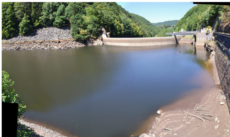
Figure 6. Vaussaire dam during low water periods. The tidal range can also be several metres under certain conditions. This exposure to atmospheric conditions can promote certain reactions (oxidation in particular) within the sedimentary matrix. [© A. Courtin-Nomade]
