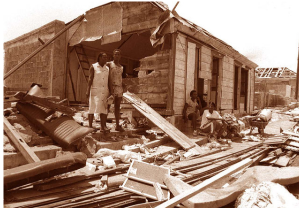
Figure 10. Damage caused by the passage of the powerful cyclone Hugo over Guadeloupe on 17 September 1989. [Source: According to http://www.guadeloupe.franceantilles.fr/actualite/education-sante-environnement/dossier-cyclone-en-guadeloupe/ ].
