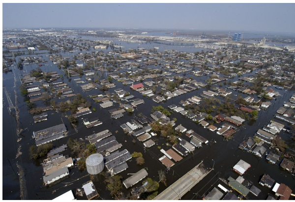
Figure 3. Flooding in New Orleans after Hurricane Katrina in August 2005.
