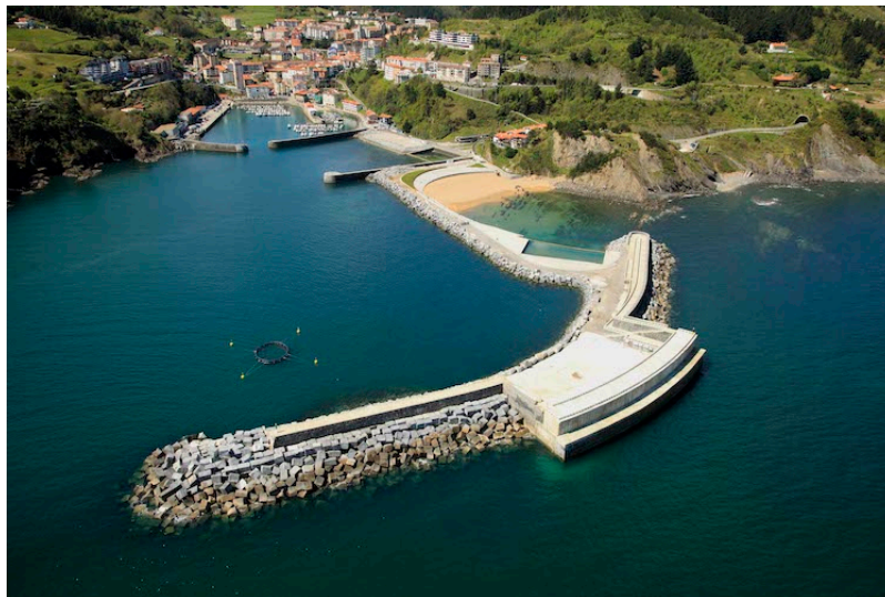
Figure 13. Mutriku wave power plant by BiMEP. www.bimep.com [Source: © Energy Agency of the Basque Government (EVE)]
