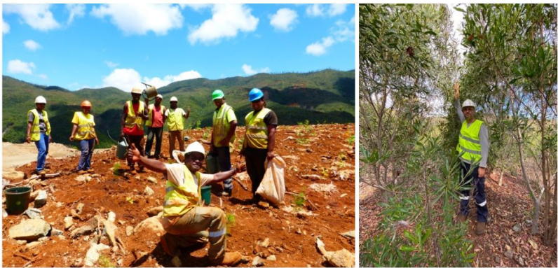
Figure 8. Six hectares of mine reclamation by phytoextraction in New Caledonia. Work carried out by the Laboratory of Bio-inspired Chemistry and Ecological Innovations (ChimEco) in collaboration with Société Le Nickel (SLN), Koniambo Nickel (KNS) and the Institut Agronomique Calédonien (IAC). They have led to the joint development of a revegetation program for barren slopes, using Ni and Mn hyperaccumulative plants. [Source: © C. Grison]
