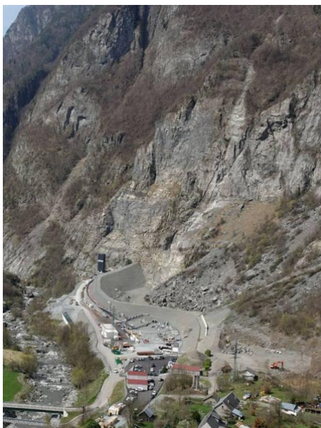
Figure 8. Merlon de protection [Source : Gavet, photo Sage]
