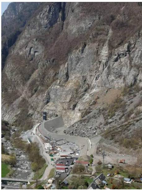
Figure 8. Protection barriers. [Source: Gavet, photo Sage]
