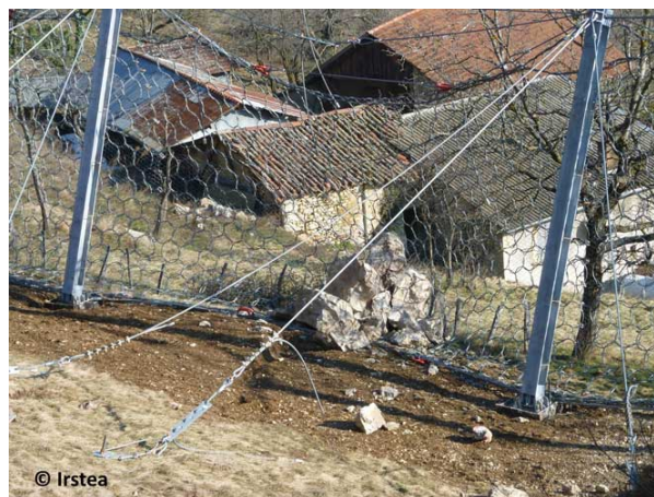
Figure 9. Deformable nets, Ripailler. [Source: IRSTEA]
