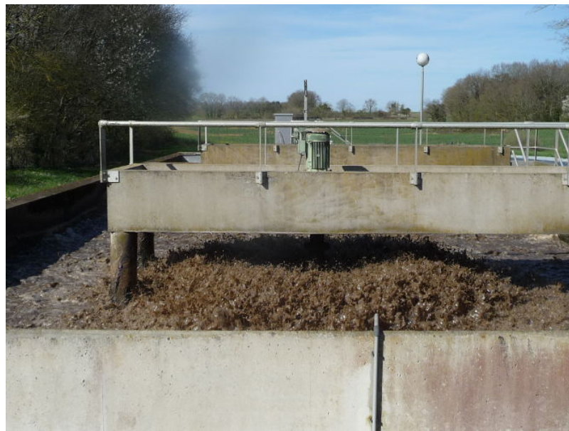
Figure 6. Activated sludge tank aerated with a mechanical agitator. [© Joseph De Laat]
