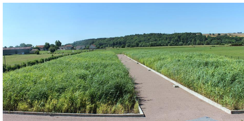
Figure 11. Filter planted with reeds. [Source: Photograph provided by Jean Voisin of the Opure group. Photos transmitted by Joelle Paing]
