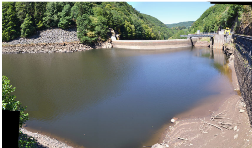
Figure 6. Vaussaire dam during low water periods. The tidal range can also be several metres under certain conditions. This exposure to atmospheric conditions can promote certain reactions (oxidation in particular) within the sedimentary matrix. [© A. Courtin-Nomade]
