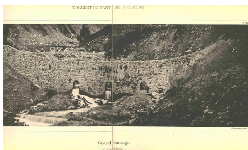
Figure 6. Grand barrage du Nant Saint Claude downstream of a landslide (73). The dam is equipped with openings allowing water to pass through until it fills with materials and thus raises the level of the stream (see Focus on slope consolidation). [© C. Kuss18]
