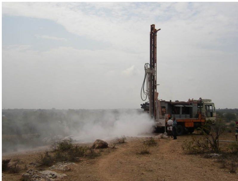
Figure 3 . Drilling in progress in a granitic aquifer using the "down the hole hammer" method. Kothur, Andhra Pradesh, India. [© B. Dewandel]
