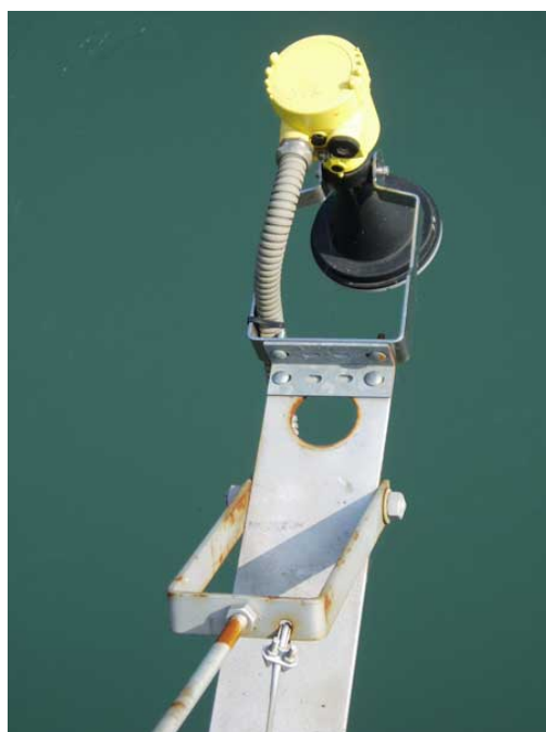
Figure 5. Level measurement by emerged radar. [© EDF DTG]
