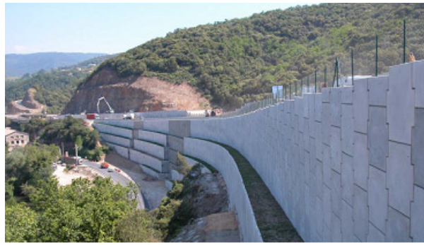
Figure 6. A high retaining wall made of "reinforced earth wall". Each wall level consists of joined reinforced concrete "scales" anchored by friction in the upstream embankment by means of metal rods. The backfill is built as the wall is erected. This technique makes it possible to create aesthetic, stable, sub-vertical and draining walls. [Source: E. Lucas, P. Sery, A. Tigoulet, D. Brancaz, 2008, Les ouvrages récents de grande hauteur en sol renforcé , Compte rendus JNGG 2008 , Nantes]
